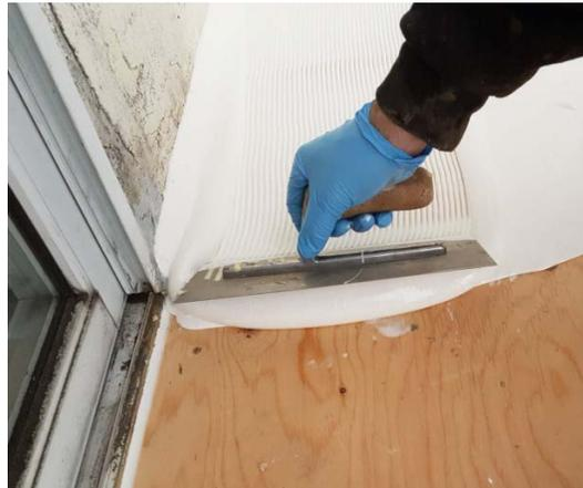
Figure 7: Spreading Base Coat
