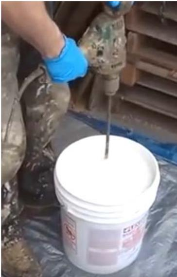
Figure 8: Mixing Base Coat
